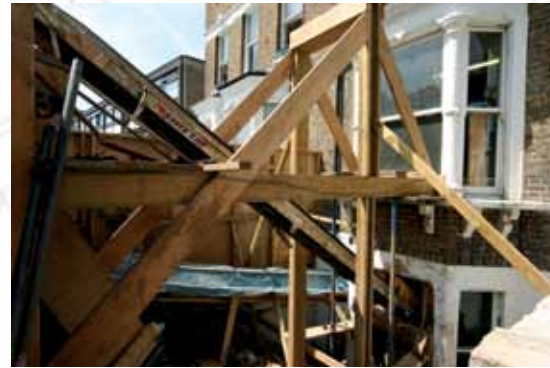
In progress: Basement dig-out.
