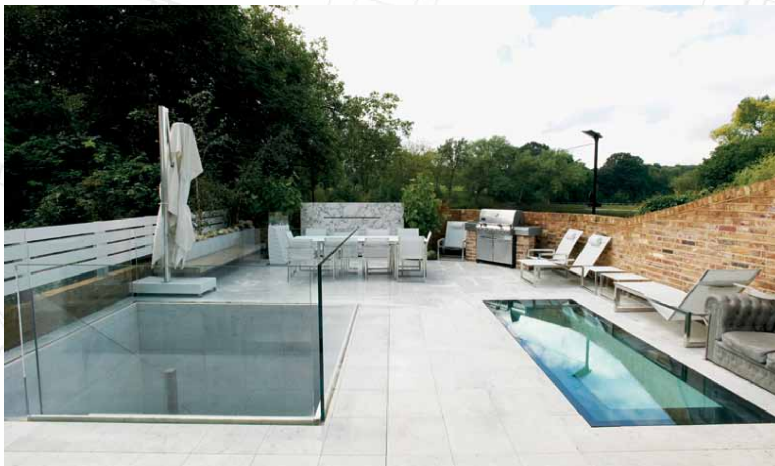
Completion: Rear patio area complete with walk on roof light above the pool in the basement.
