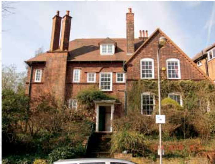
Before: Original structure.
